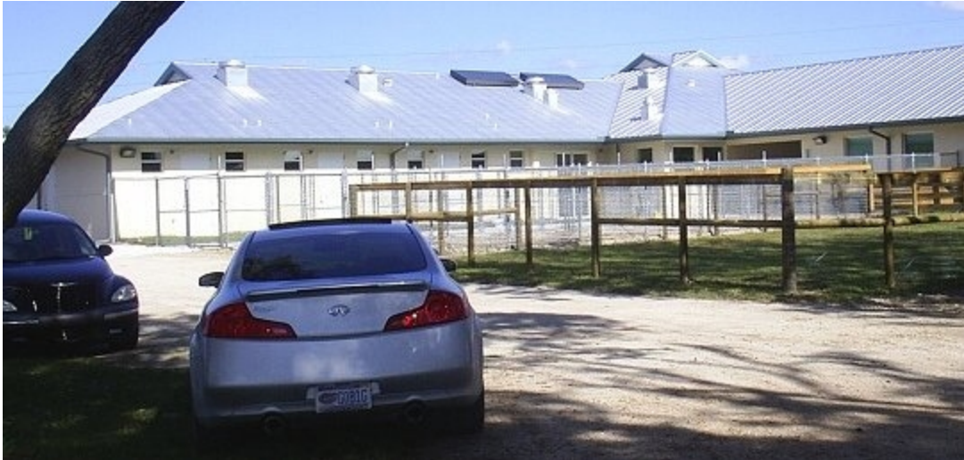
Rear Exterior of the Clinic showing two Solar Panels for Water Heating mounted to a Heat Reflecting Roof.
