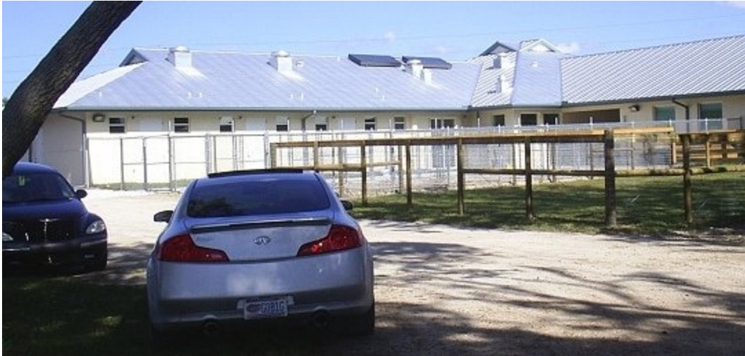
Rear Exterior of the Clinic showing two Solar Panels for Water Heating mounted to a Heat Reflecting Roof.
