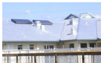
2 Passive Solar Water Heating Panels on a heat reflecting roof.
