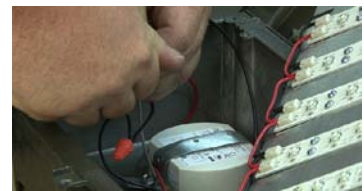
FIGURE 4: Connecting the LED driver wires to the LED light bulb.
