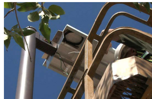
FIGURE 3: Attaching solar panel to pole.
