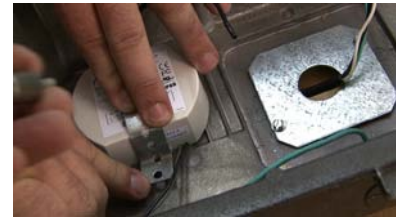
FIGURE 2: Installing the LED driver into the wall pack fixture housing.
