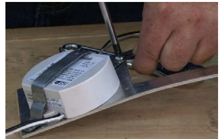
FIGURE 2: Installing the LED driver onto the diffuser.
