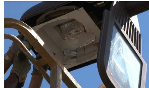
FIGURE 1: Opening cover for parking lot fixture to remove reflector and electrical components
