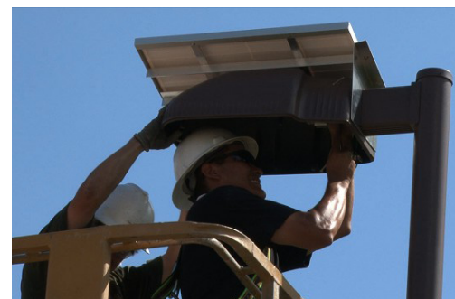
FIGURE 4: Attaching the fixture to the pole.
