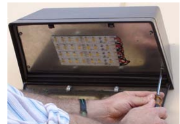
FIGURE 5: Screwing the light bulb into the wall pack housing.
