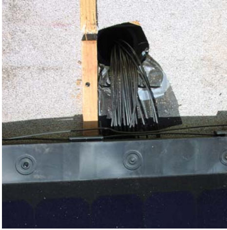
A penetration point for homeruns – before and after flashing
