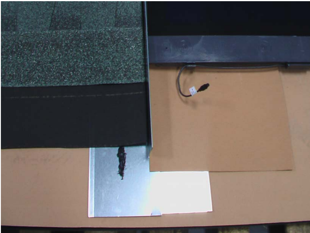
Typical T Flashing installed as transition between composition shingles and SolarSave™
