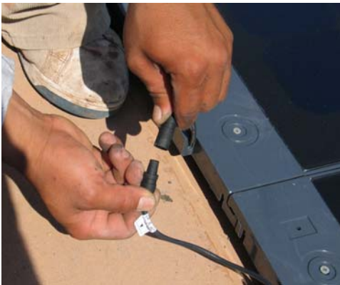
An MC connector completing a series connection
